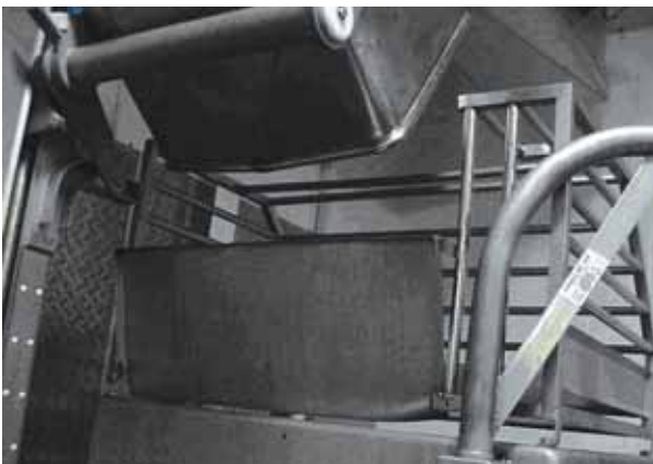
Grinder hopper fenced to accommodate bin lift with extension to reach distance under the bin
