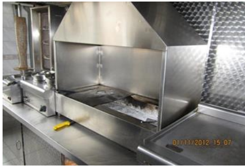
Custom made Grill with 'funnel' enclosure
